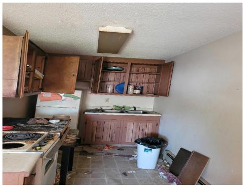
**Photo 4:** View of positive vinyl sheet flooring 2 layers in building 211 2<sup>nd</sup> floor south end apartment kitchen.
