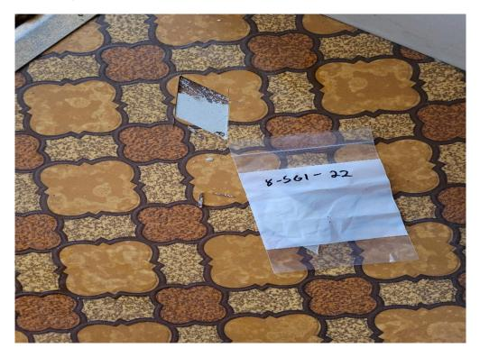
**Photo 3**: View of positive vinyl sheet flooring in building 211 2<sup>nd</sup> floor north end apartment kitchen.
