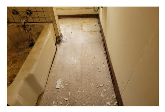
**Photo 5**: View of positive vinyl sheet flooring in bathroom of building 213 2<sup>nd</sup> fllor apartment.
