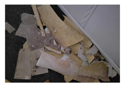
**Photo 8**: View of positive vinyl sheet flooring debris pile in building 211 1<sup>st</sup> floor west side office located in middle room and under carpet and shower.
